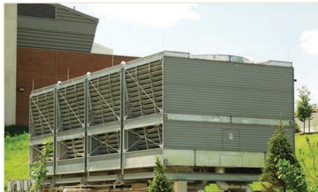
PHOTO 1 Four cell crossflow open circuit cooling tower.
