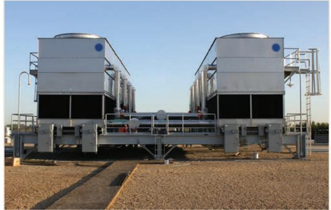
PHOTO 2 Multi-cell counterflow open circuit cooling tower installation.
